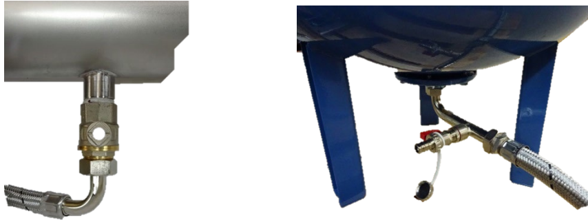
Fig 2.3a & b Isolation valve on system pipework & Drain cock on vessel.
